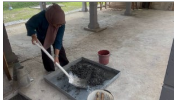
Rajah 2: Manual mixing of concrete materials during the concrete preparation process.
