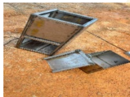
Rajah 2: Welding and assembly of the Spin Compost Mini main structure
