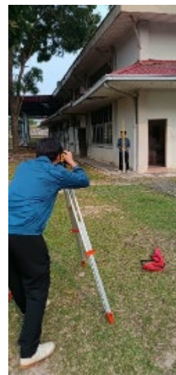
Rajah 2: Soil Levelling Investigation Work
